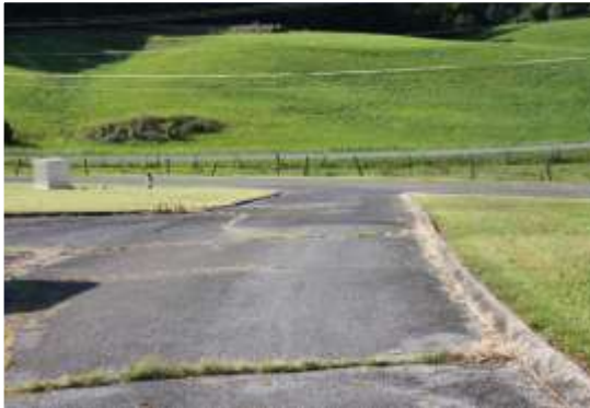
ASPHALT ENTRY DRIVE
